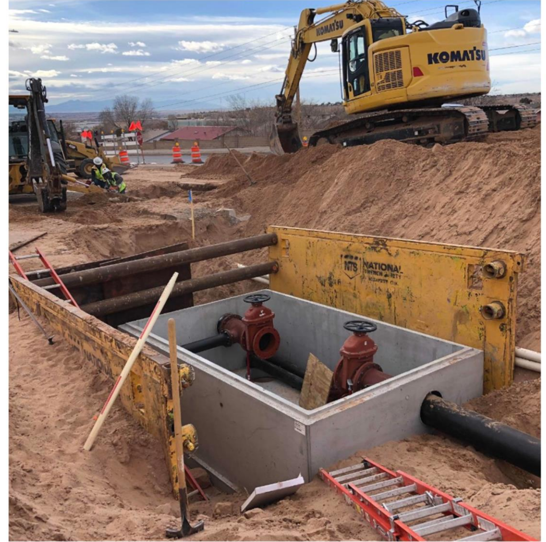
City of Rio Rancho Road Project
