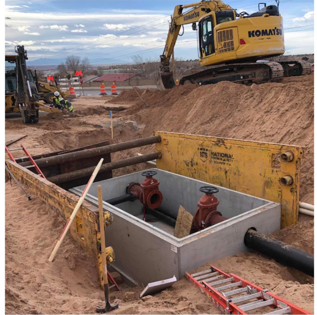
City of Rio Rancho Road Project
