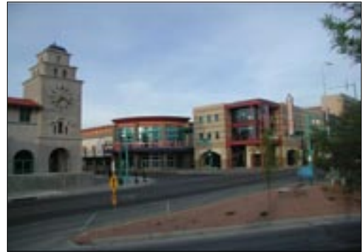
Phase I of the Alvarado Multi-Modal Transportation Center at 1 st and Central in downtown Albuquerque with Phase II under construction to the south.
